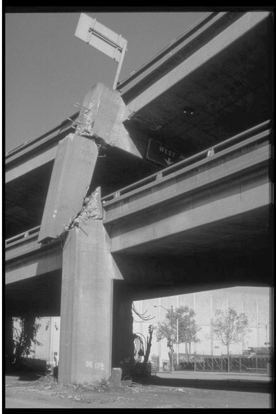
Figure 3.3: This damaged column from a section of the Cypress Viaduct that did not completely collapse illustrates the failure of the joint at the level of the lower roadway, which engineers agreed was the main cause of the disaster. Source: Loma Prieta Collection, Earthquake Engineering Research Center, University of California, Berkeley.
