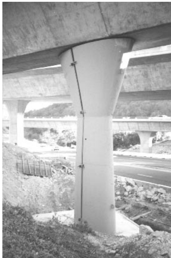
Figure 2.10: Steel shell in position around column, ready for welding and grouting. Photograph by the author.
