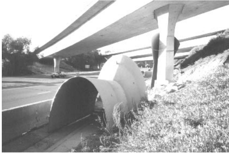
Figure 2.9: Steel shell prior to installation, intersection of State Route 52 and Genesee Avenue, San Diego. Note irregular shape to fit around hexagonal flared columns, seen in background. Photograph by the author.
