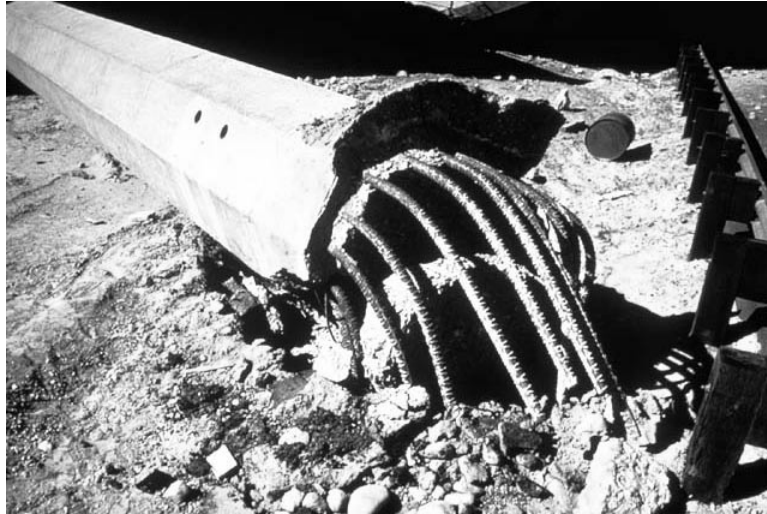
Figure 2.3: Close-up of column from Figure 2.2, showing that failure was caused by column reinforcement pulling out of the footing. Source: Godden Collection, Earthquake Engineering Research Center, University of California, Berkeley.
