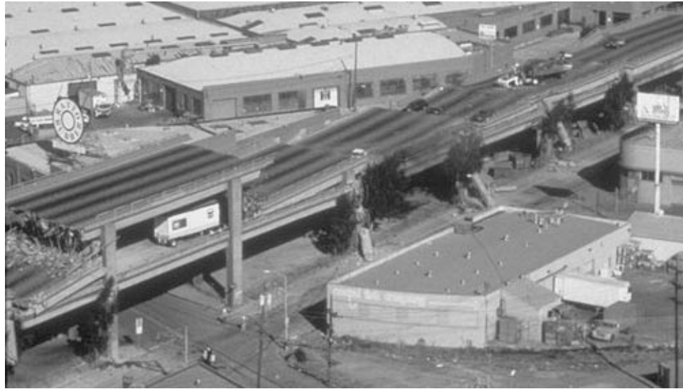
Figure 3.1: Part of the collapsed portion of the Cypress Viaduct in Oakland following the Loma Prieta Earthquake. Source: Loma Prieta Collection, Earthquake Engineering Research Center, University of California, Berkeley.
