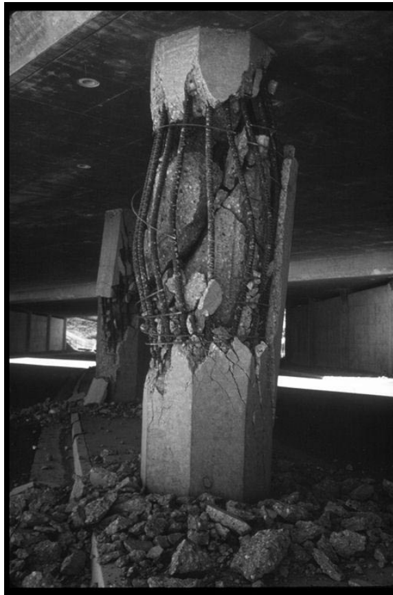
Figure 2.4: Column damage to another structure at the I-5/I-210 interchange, 1971 San Fernando earthquake, caused by rupture of horizontal reinforcement hoops. Source: Steinbrugge Collection, Earthquake Engineering Research Center, University of California, Berkeley.
