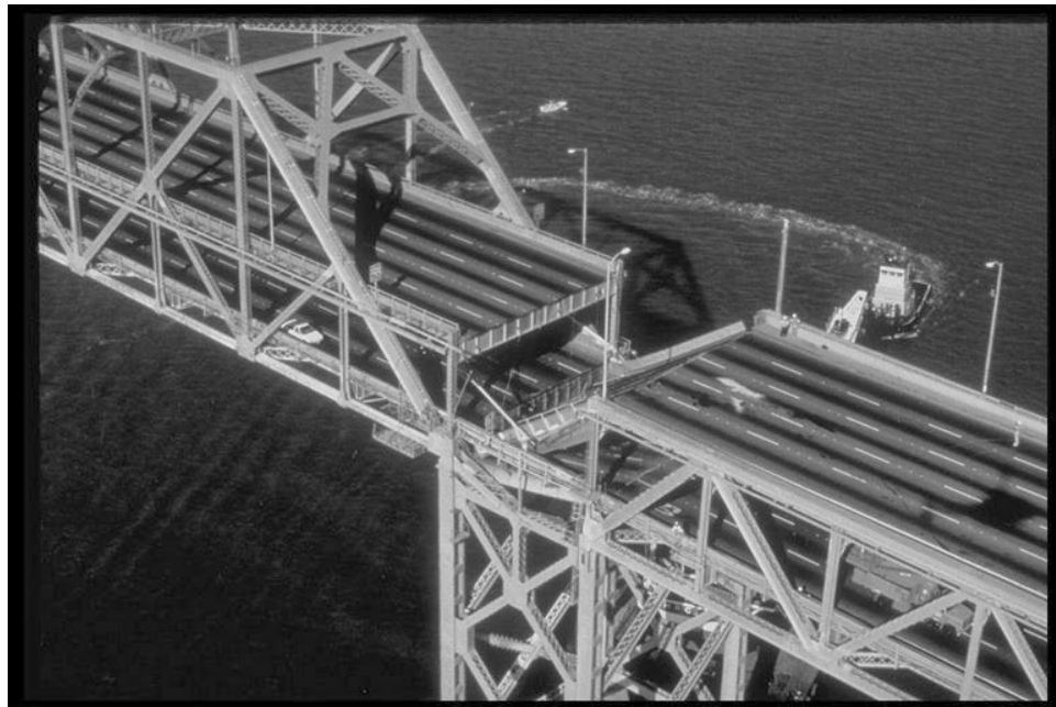
Figure 3.2: Collapsed deck segment of the San Francisco-Oakland Bay Bridge after the Loma Prieta earthquake. Source: Loma Prieta Collection, Earthquake Engineering Research Center, University of California, Berkeley.
