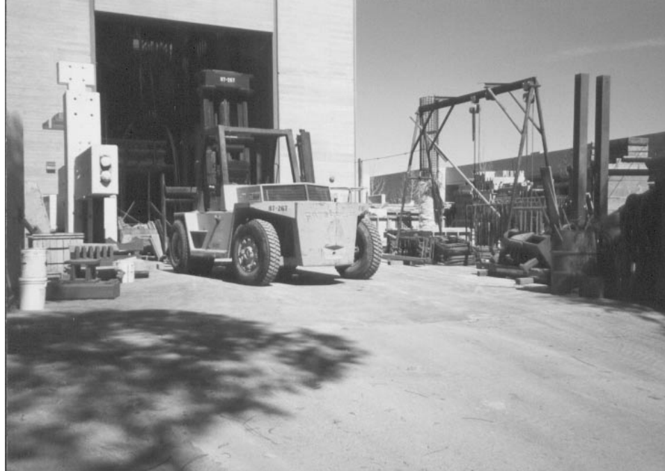
Figure 6.1: An exterior view of one of the main buildings of the Structures Lab. Photograph by the author.
