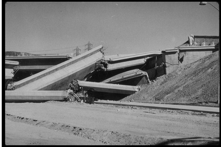
Figure 2.2: Collapse of bridge at I-5/I-210 interchange, 1971 San Fernando earthquake, showing fallen columns (foreground) and segments of bridge deck. Source: Steinbrugge Collection, Earthquake Engineering Research Center, University of California, Berkeley.
