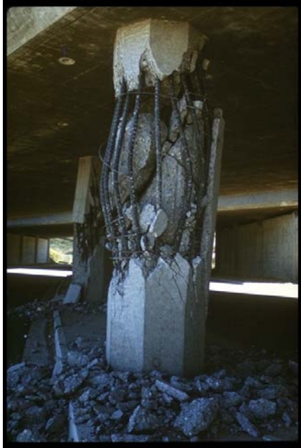
Figure 2. Column damage caused by rupture of horizontal reinforcement hoops. Source: Steinbrugge Collection.
