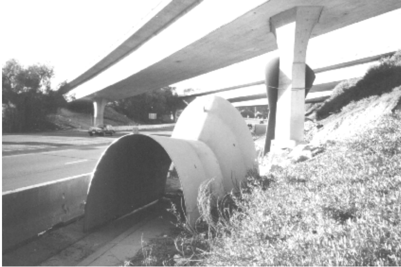
Figure 4. Steel shell prior to installation, intersection of State Route 52 and Genesee Avenue, San Diego. Note irregular shape to fit around hexagonal flared columns, seen in background. Photograph by the author.
