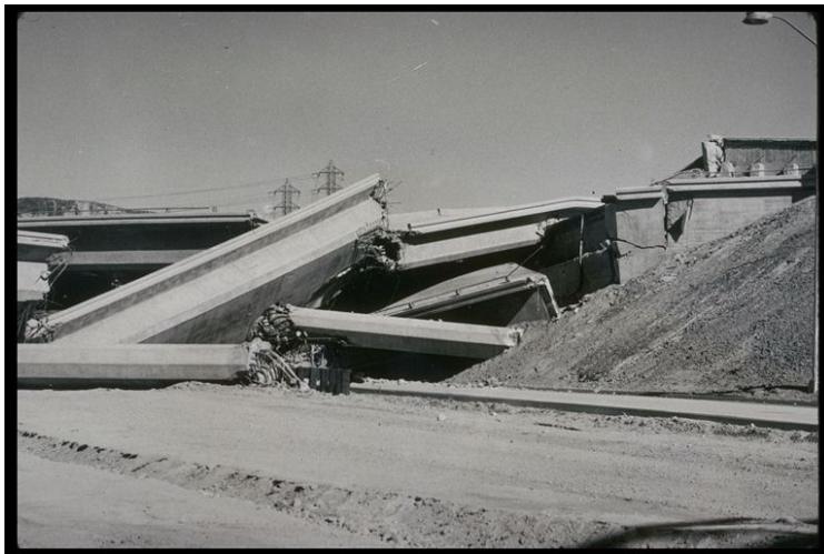
Figure 1. Collapse of bridge at I-5/I-210 interchange, 1971 San Fernando earthquake. Source: Steinbrugge Collection, Earthquake Engineering Research Center, University of California, Berkeley.
